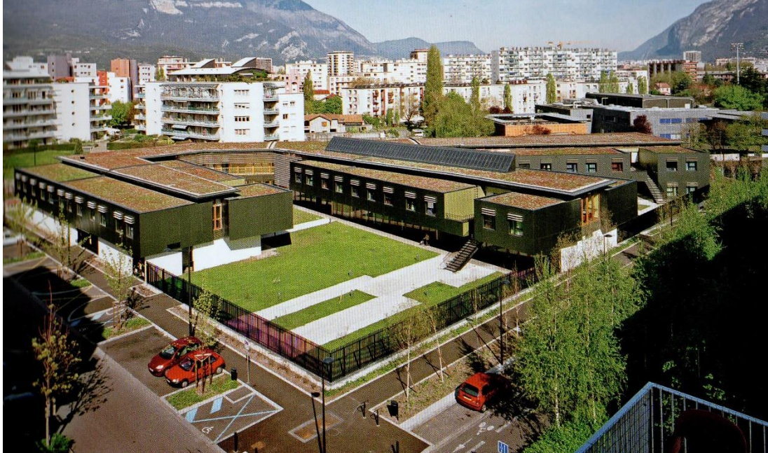
Figure 3. 15 The integration of two gardens between the three building blocks in EHPAD Vigny-Musset, Grenoble, France.
