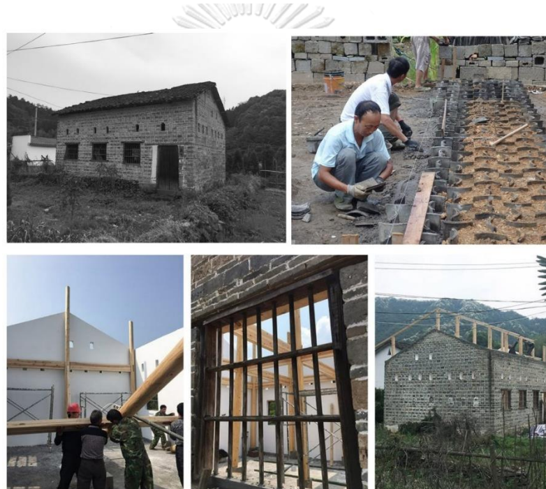
Figure 3. 10 Qi Men Black Tea House in different construction stages (魏唐辰希, 2018).
