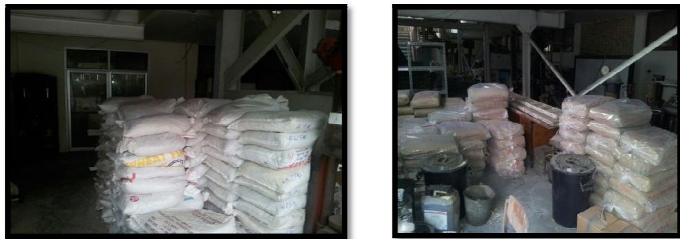
Figure 3.1 Materials (sand, gravel and cement)
