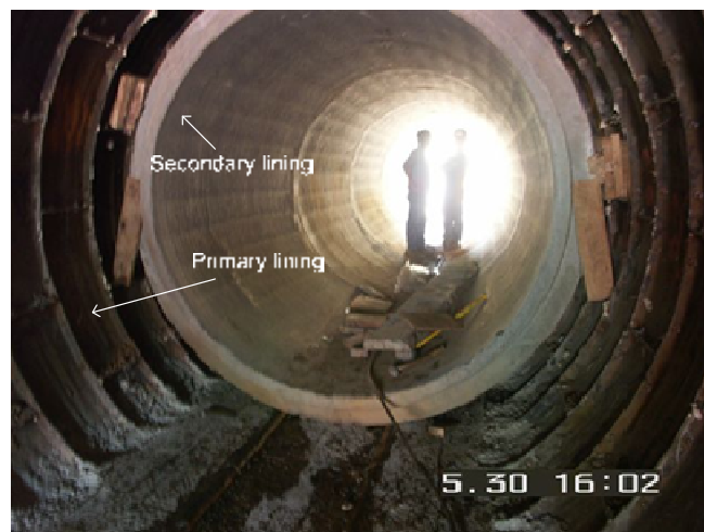
Figure 2.2 Primary lining and secondary lining
