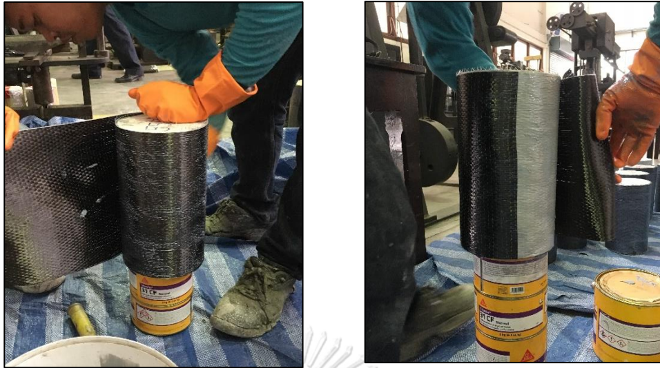
Figure 4.17 FRP wrapping procedures
