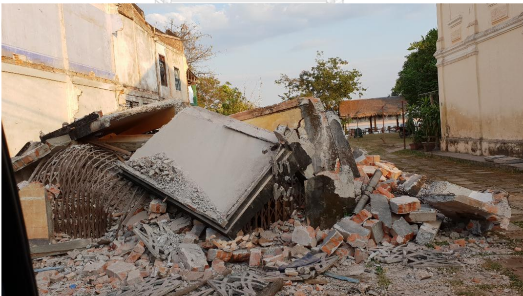
Figure 42 Unauthorized demolition of terraced house in Champasak town
