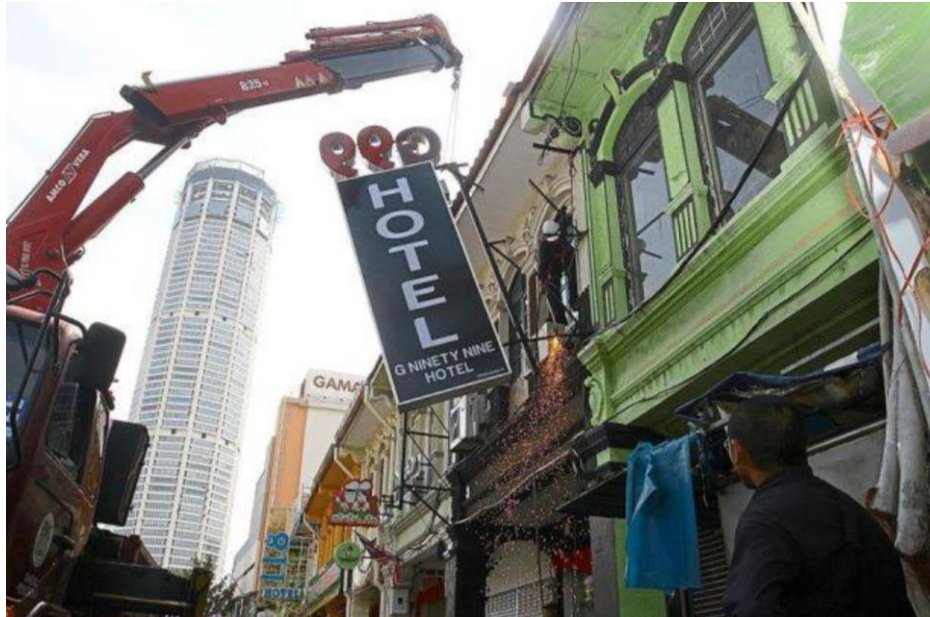
Figure 54 Hotel demolition in process
