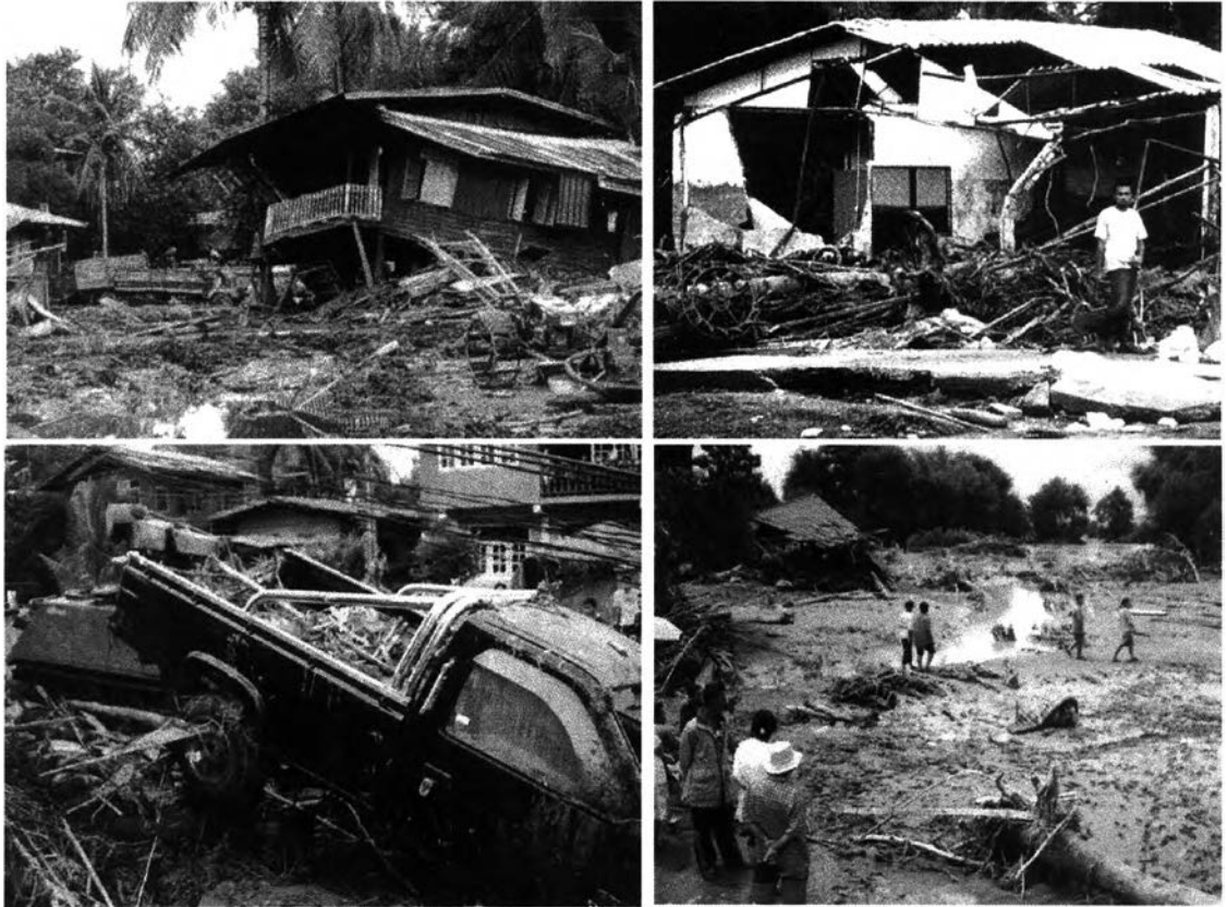
Figure 6-6 Four photographs showing some examples of seriously structural damage of houses and other infrastructures in Ban Nam Ko Yai (in the area between A and B in Figure 6-5) battered and caused by the fast-moving 8/11 flow-flood.
