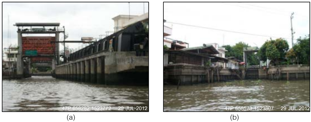
Figure 2-4 (a) Main floodgate and pump at the Chakphra Canal, and (b) dyke along the Chakphra Canal with the floodgate at the Jaoarm Canal
