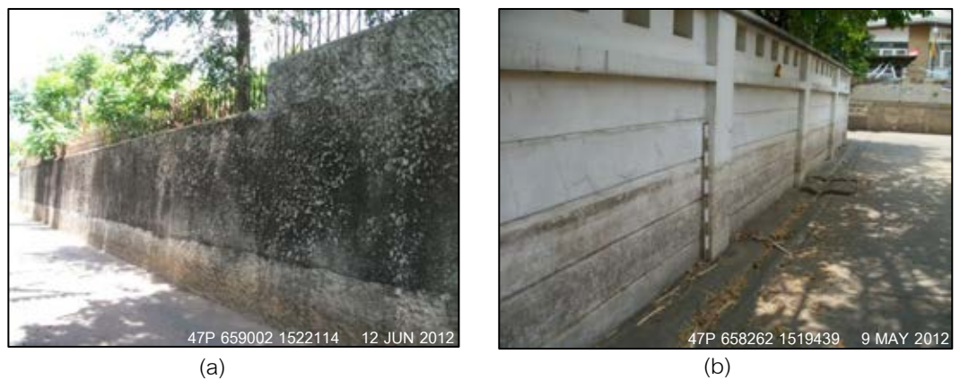
Figure 2-6 Traces of flood near (a) the Bangkhunnon Canal and (b) the Wat Deedud Canal
