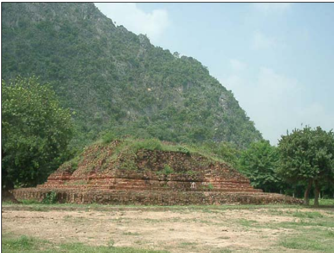
Figure 4.3 General view of Thungsetthi monument after restoration.
