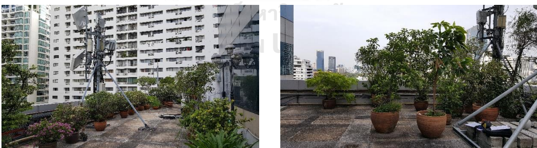
Figure 6A Green roof on SG Tower Building (SGT)
