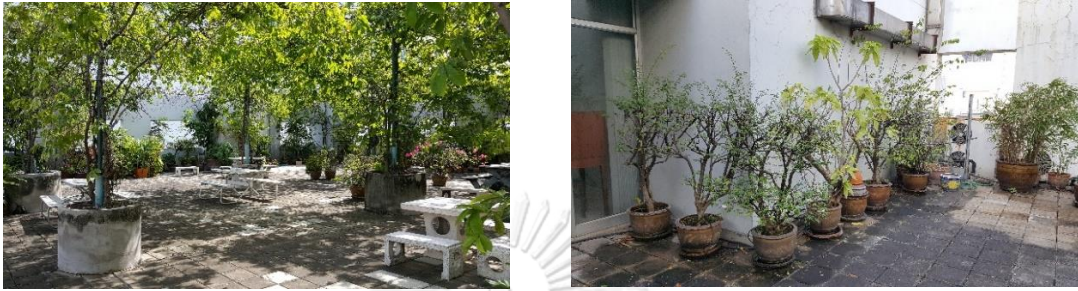
Figure 7A Green roof on 60th Anniversary Building at Faculty of Veterinary Science (SXV)
