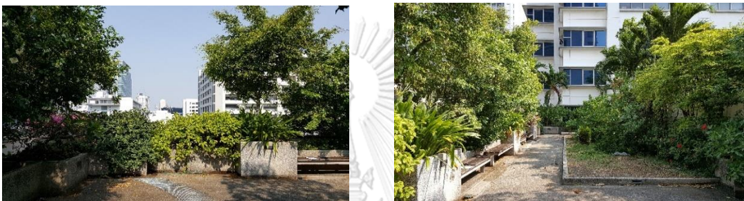
Figure 1A Green roof on Aor Por Ror Building (APR)
