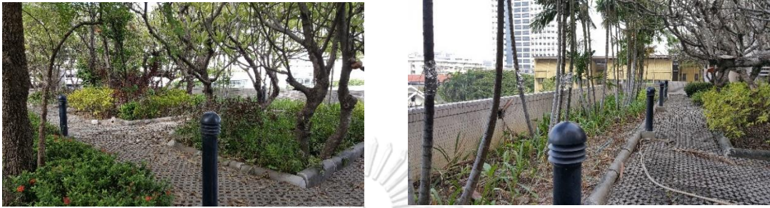
Figure 3A Green roof on Mahitaladhibesra Building (MHT)
