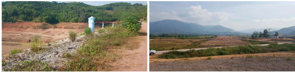
Hin River Reservoir
