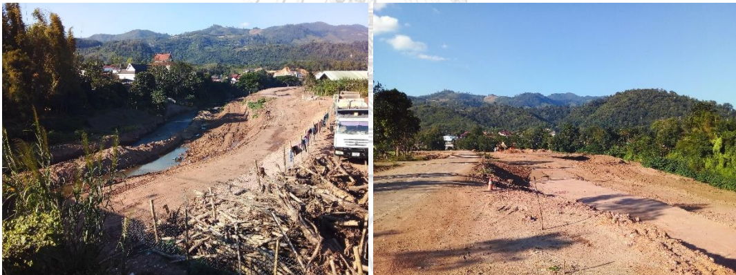
Figure 7.7: Clearance works for erosion and flood protection construction.
