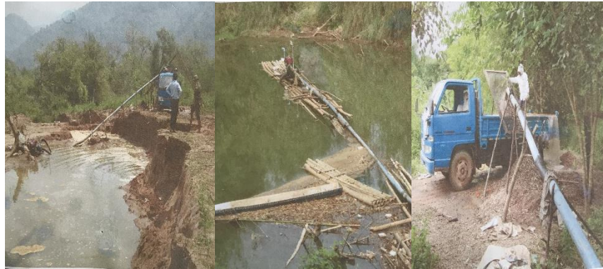
Figure 6.24: Excavate the sand, gravel, and minerals along the Kor River.
