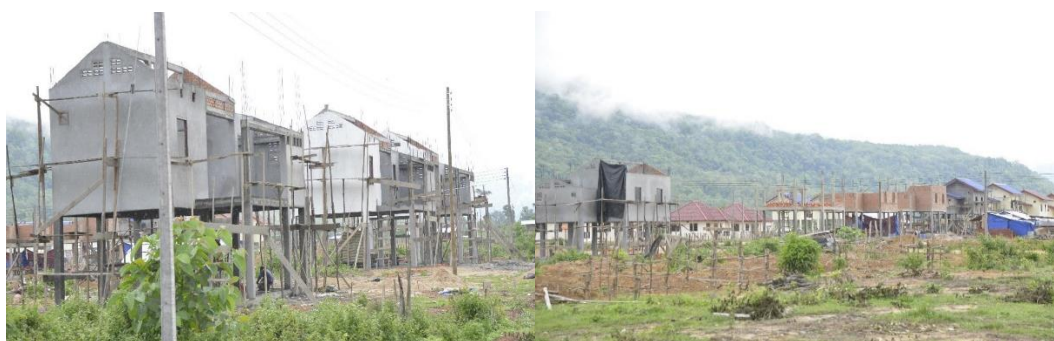
Figure 6.31: new elevated houses
