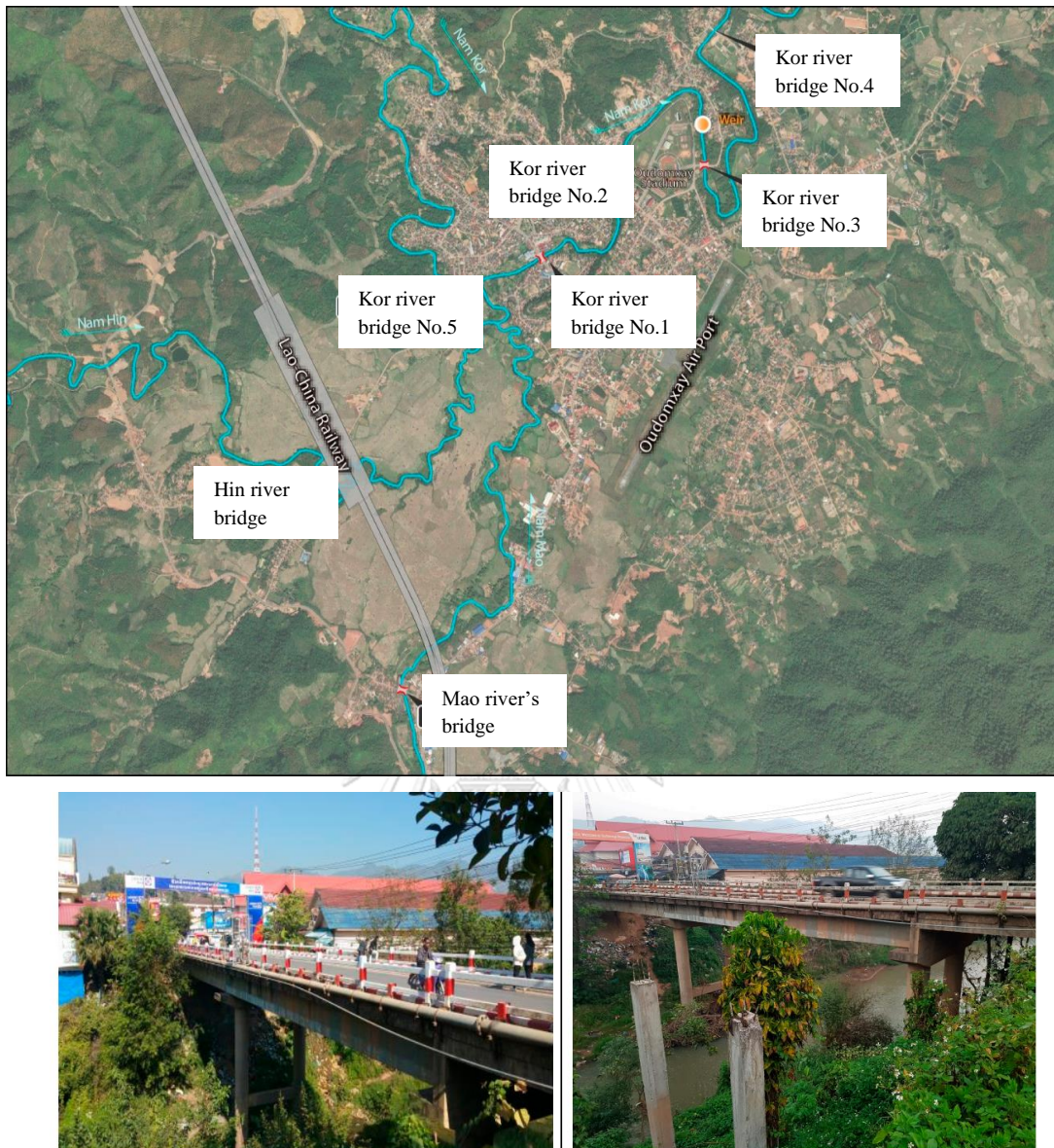
Figure 7.16: A sample of Kor River Bridge No.1
