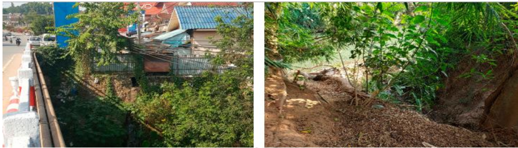
Drainage Outlet near the Market
