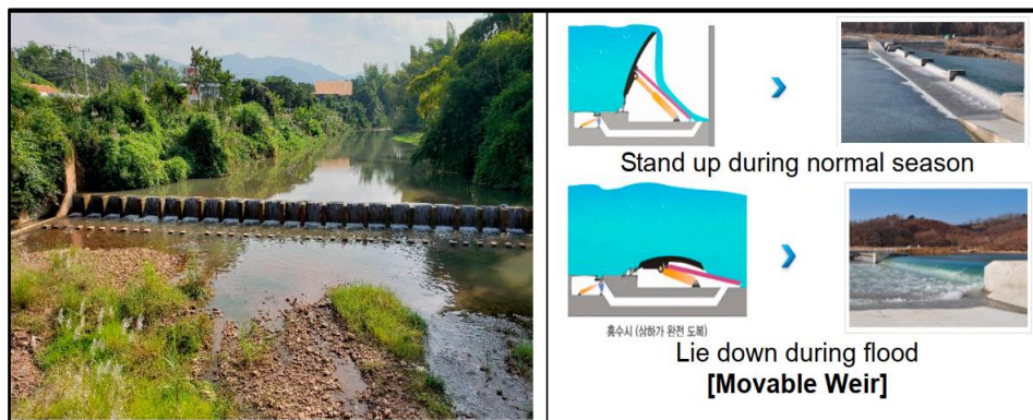
The existing Mao River weir
