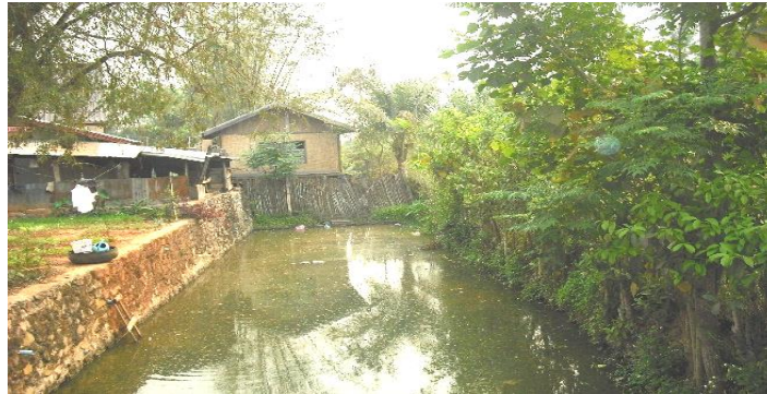
Figure 5.4: Existing drainage system
