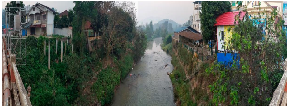
Figure 4.20: Present condition at the downstream of Kor River Bridge 1.
