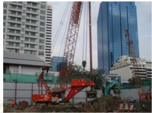
b) drilling by auger &amp; bucket
