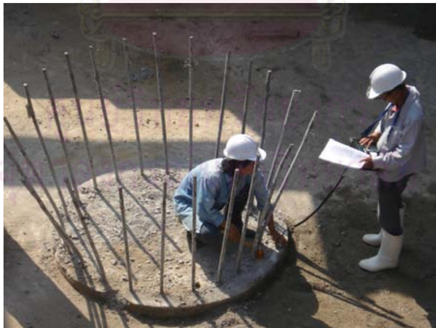
Figure 3.13 Pile integrity recorded with Sonic integrity/seismic test
