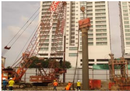
a) Install casing
