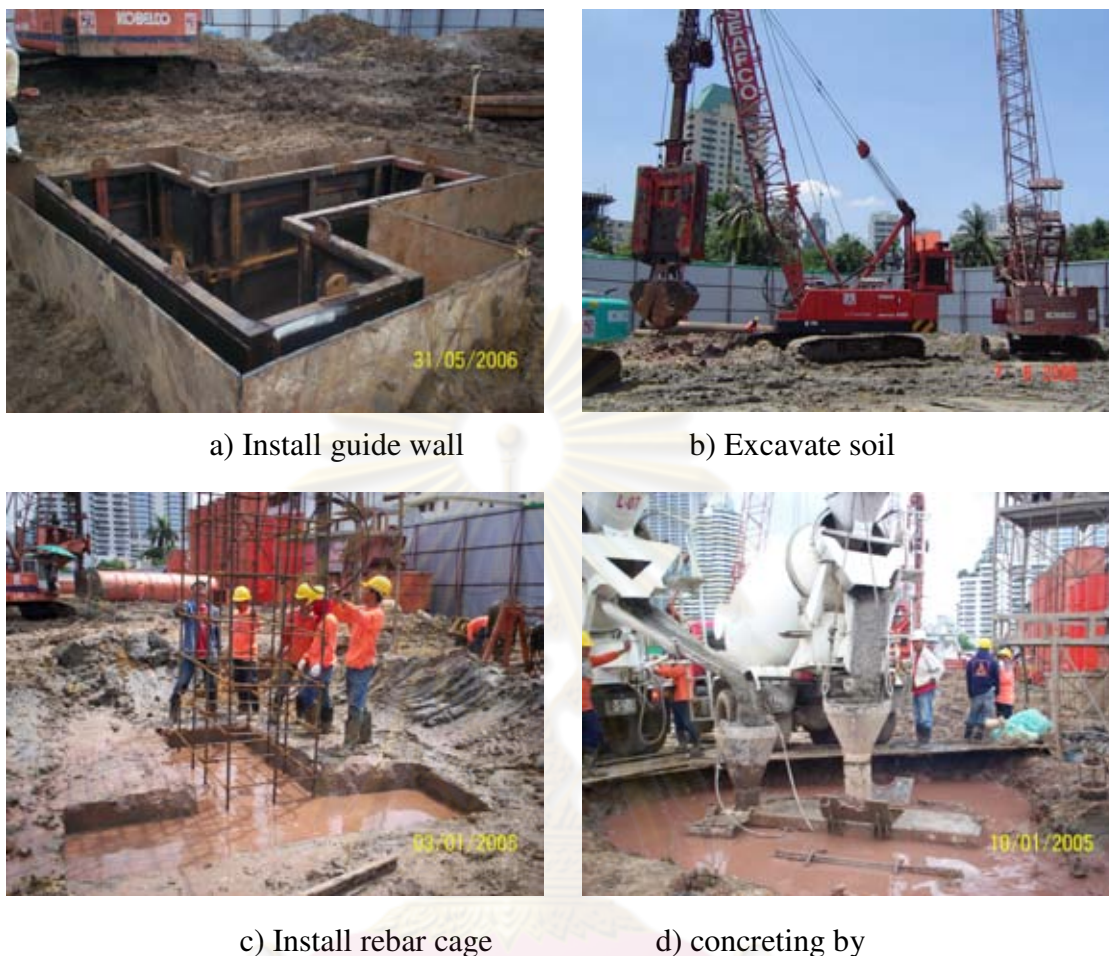
Figure 3.11 Construction sequence for T-shape barrette
