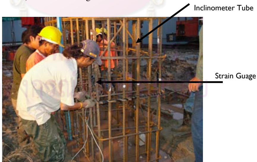
b) Geotechnical Instruments during installation
