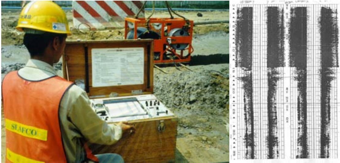
Figure 3.12 Trench profile recorded with drilling monitoring/Koden equipment
