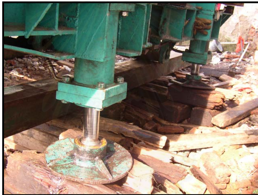
Figure 4.21 Jack equipment of pushing-machine which use hydraulic power
