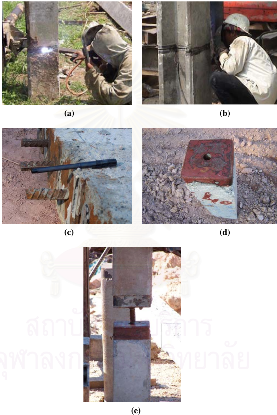
Figure 4.23 Joining system of Thai I-shape piles (a) and Indonesian triangle piles (b), and steel rebar anchor (c), special pile's cap (d), and its connection process (e) of Malaysian rectangular pile.
