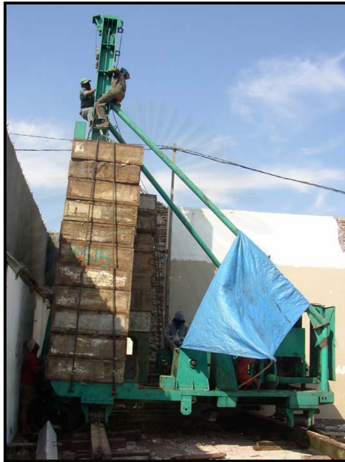
Figure 4.17 Indonesian pile-driving machines
