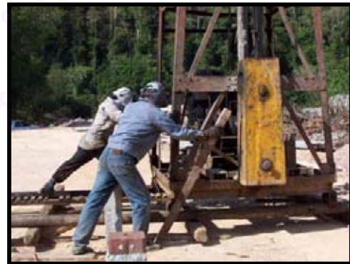
Figure 4.13 Mechanism of shifting an support which relies on man power at Malaysian drop-hammer
