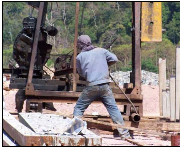
Figure 4.15 Mechanism of backward movement of Malaysian drop-hammer
