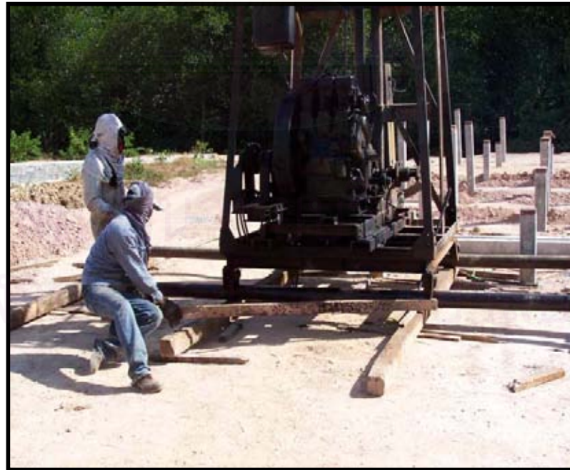
Figure 4.8 The jacking mechanism of Malaysian drop-hammer
