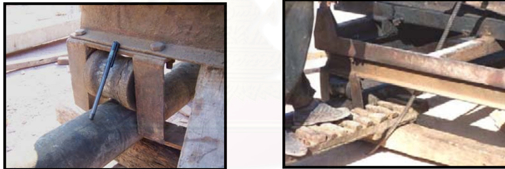
(a) The steel pipe and wheel
