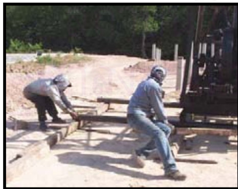
Figure 4.13 Mechanism of shifting an support which relies on man power at Malaysian drop-hammer
