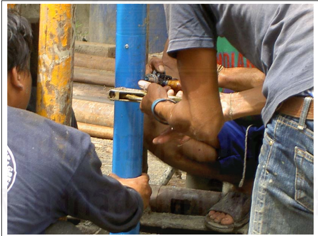
Figure 3.34 Process of rivet installation
