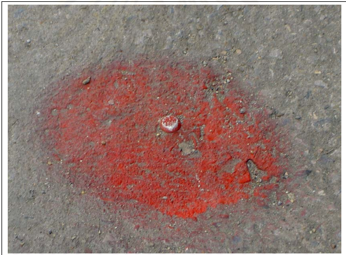
Figure 3.21 Upper end of steel rod
