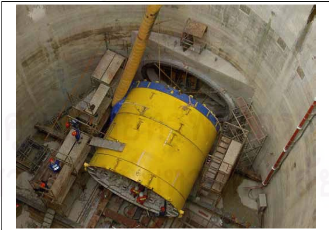
Figure 3.3 The assembly of TBM machine
