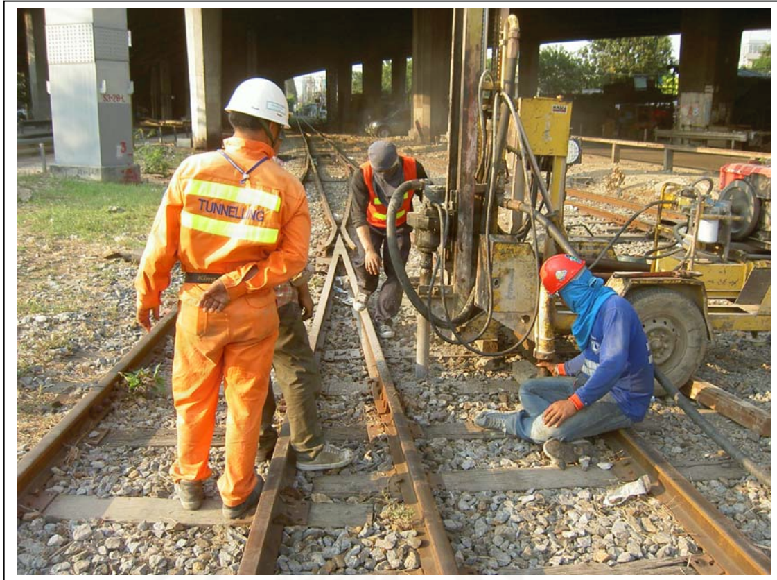
Figure 3.23 Installation of settlement point
