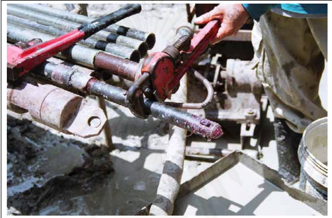
Figure 3.26 Coupling and anchor of deep settlement point
