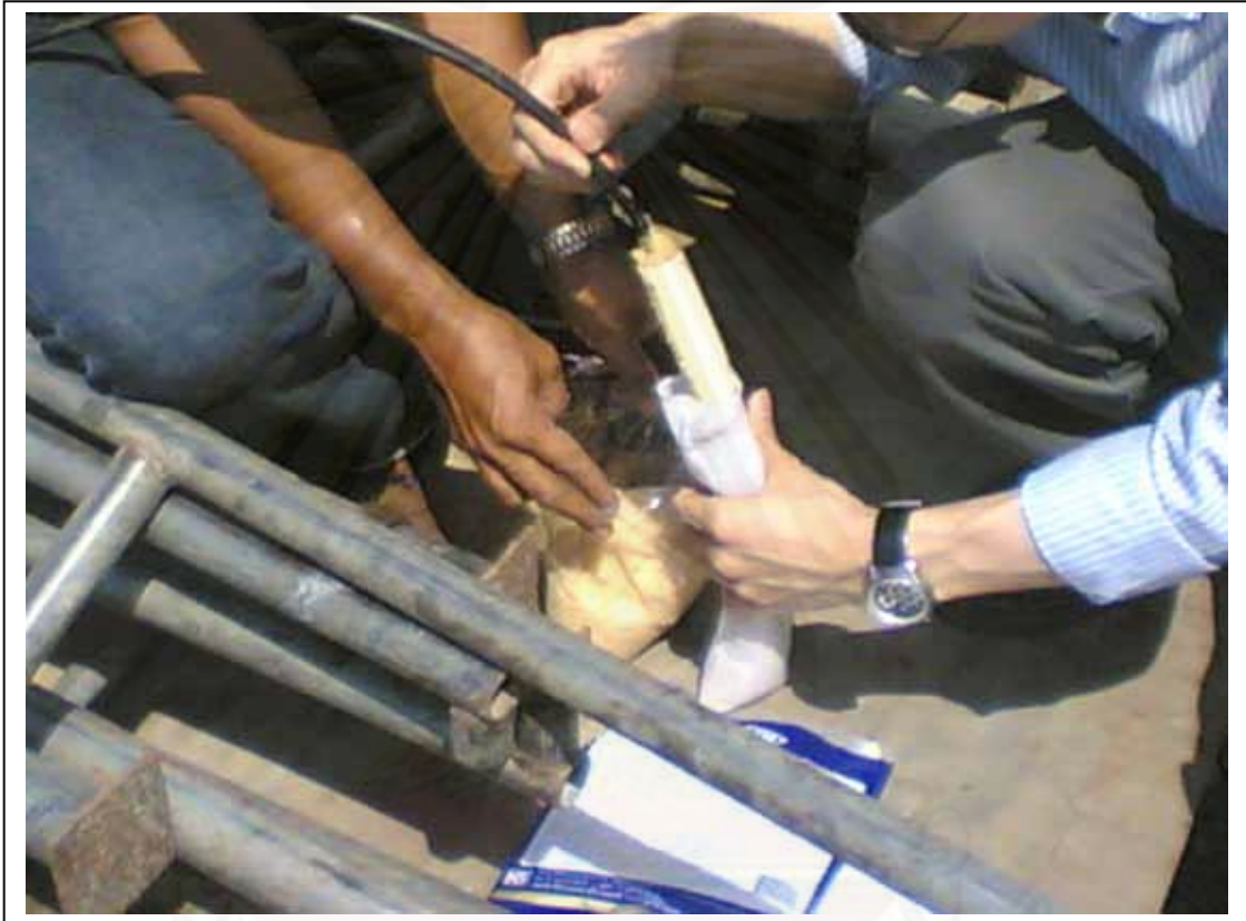
Figure 3.37 Piezometer probe and sand bag
