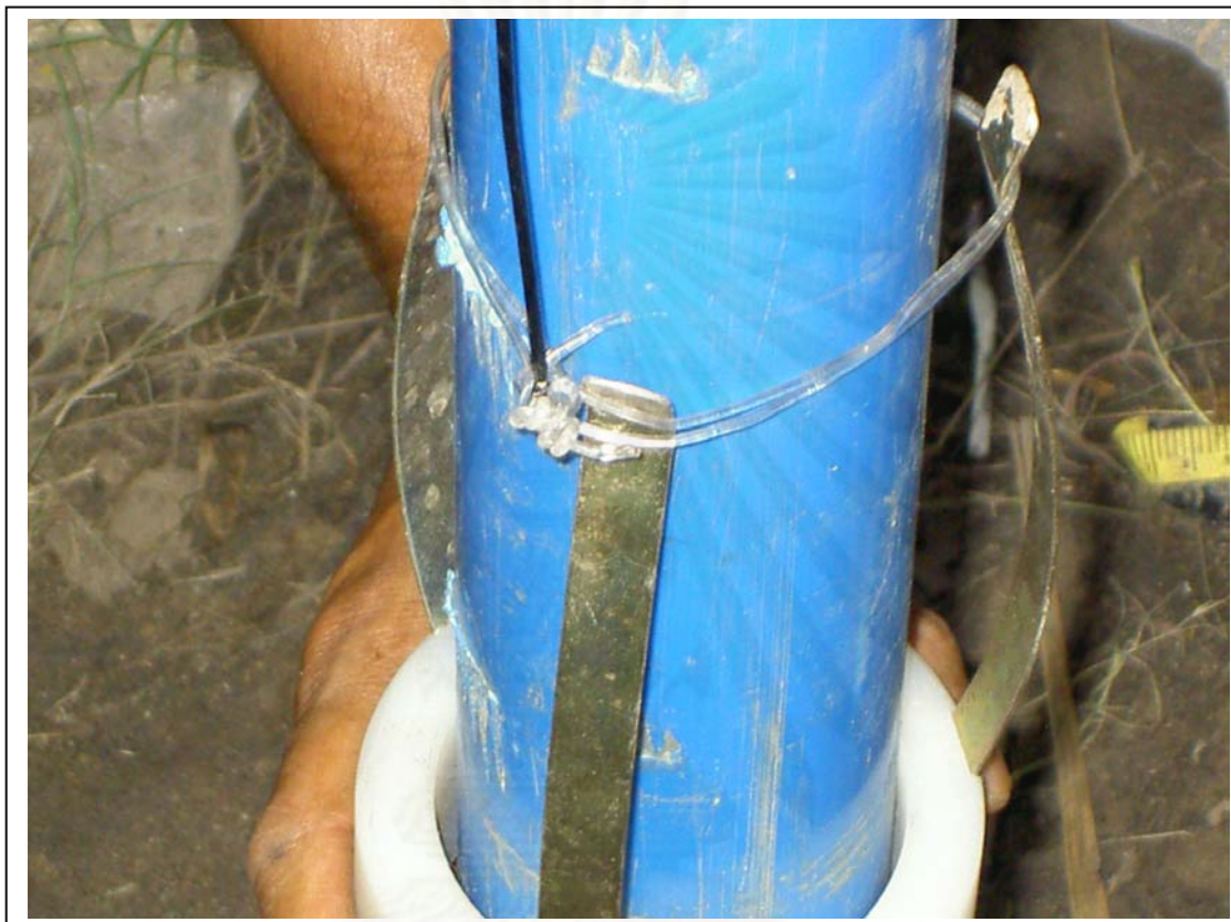
Figure 3.30 Detail of compression wire
