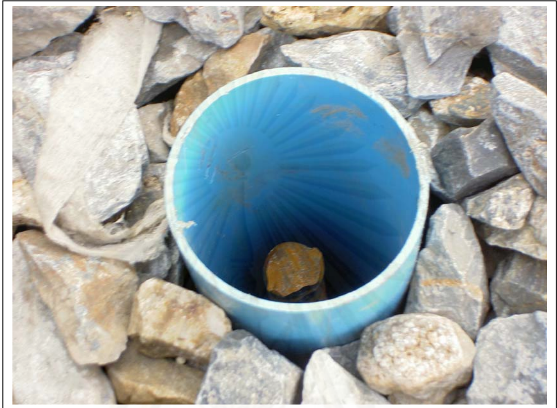
Figure 3.24 Settlement point after installation
