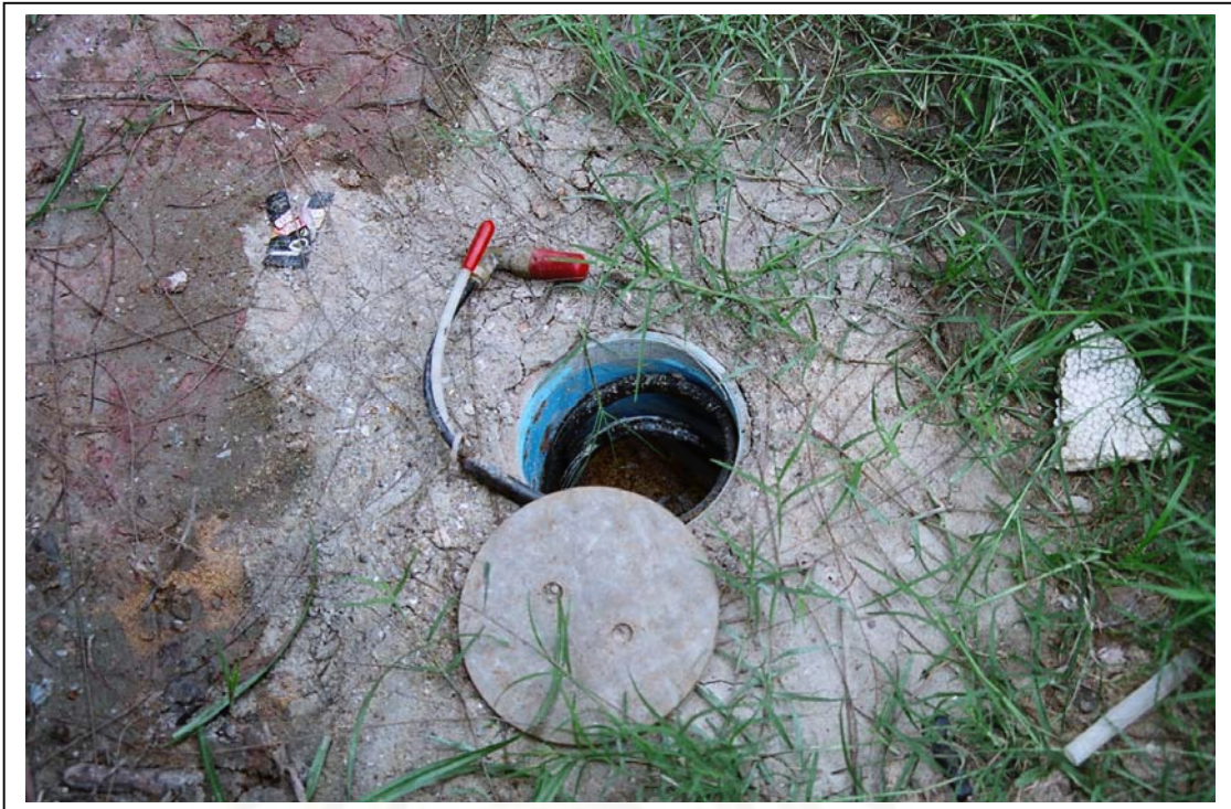
Figure 3.39 Protection cap of piezometer
