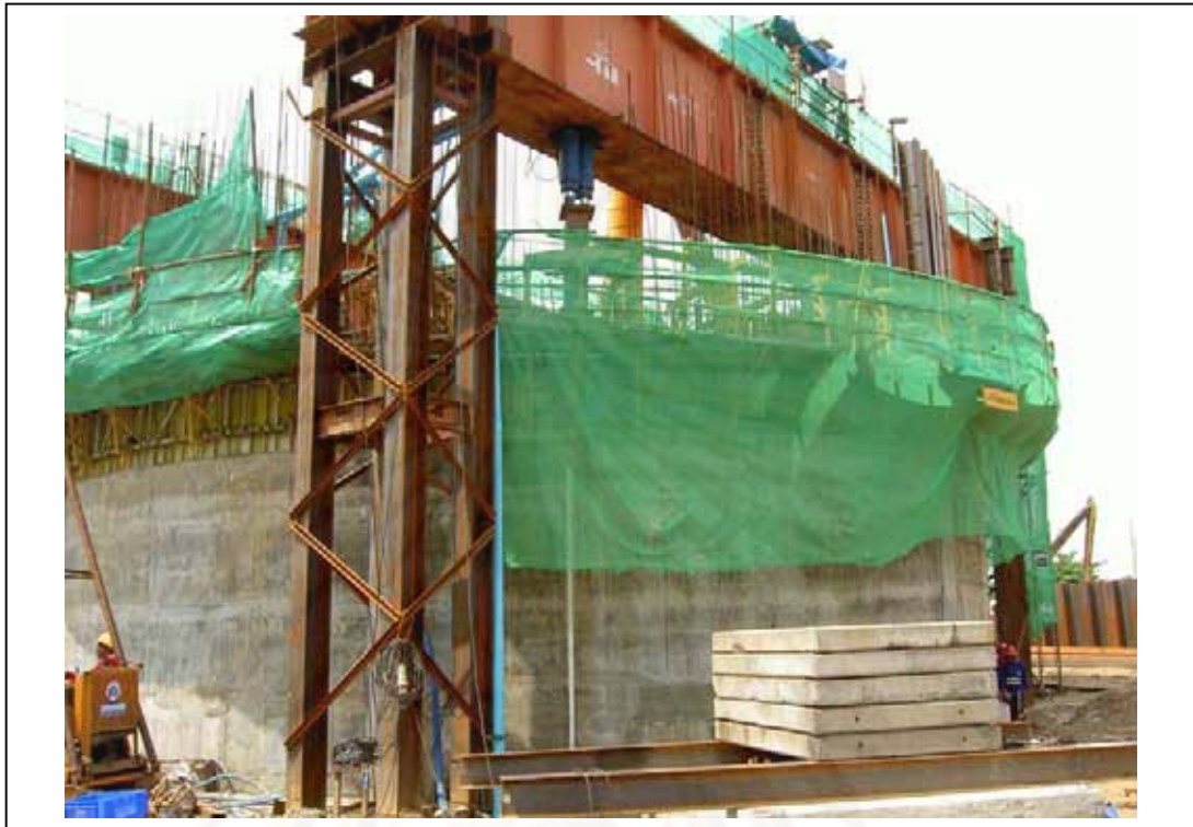
Figure 3.2 Photo of sinking shaft at Wat Chong Lom
