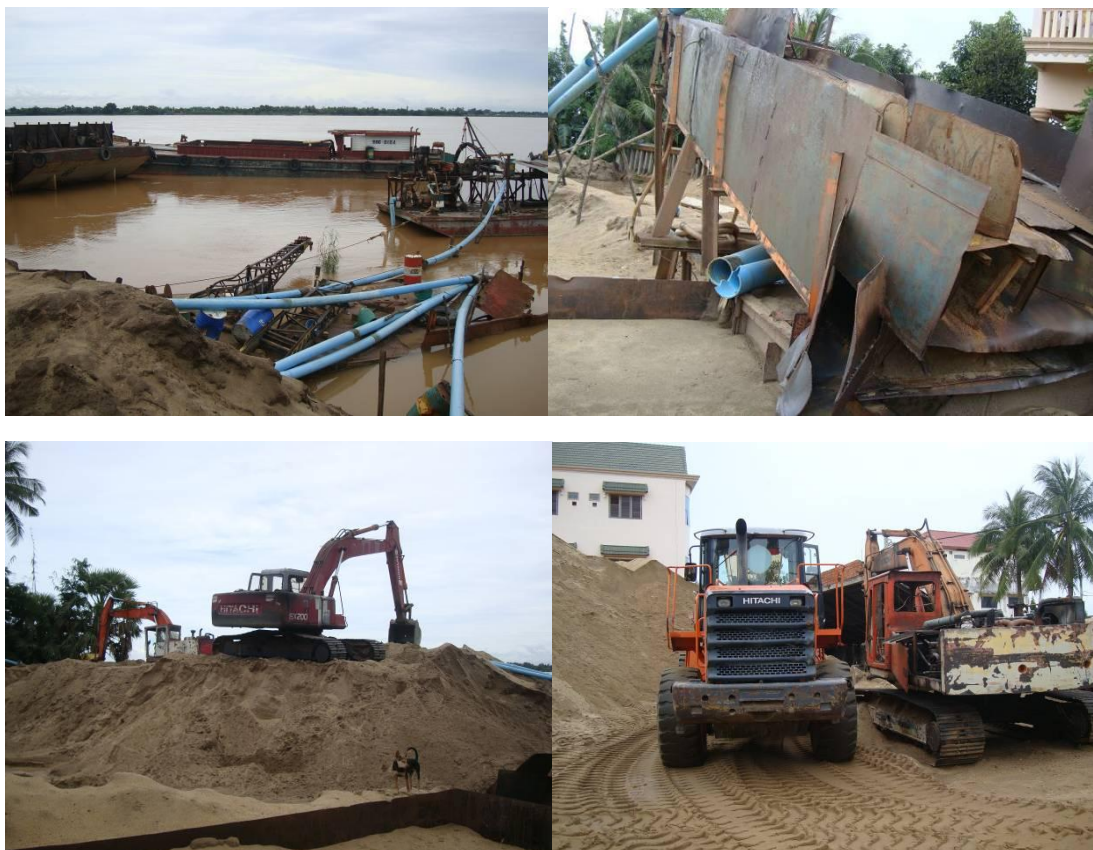
Figure3.1 Location of site investigation
