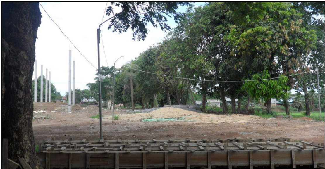
Photograph 6: Construction work in the pagoda
