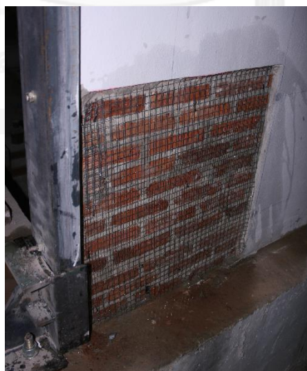
Figure 3-11. Reinforcement at the corners of infill panel
