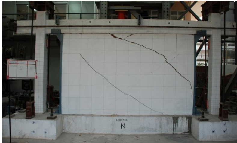
Figure 4-47. Retrofitted specimen MIRCF02 at LS Performance Level
