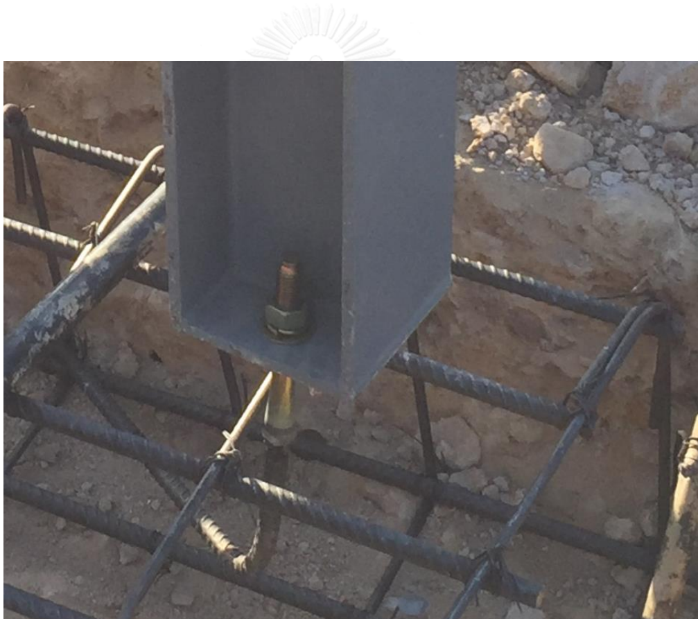
Figure 3.1-4 Steel hook embedded in the foundation
