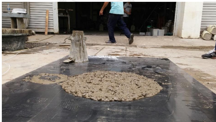
Figure 3.2-2 Pre-mix slump flow check
