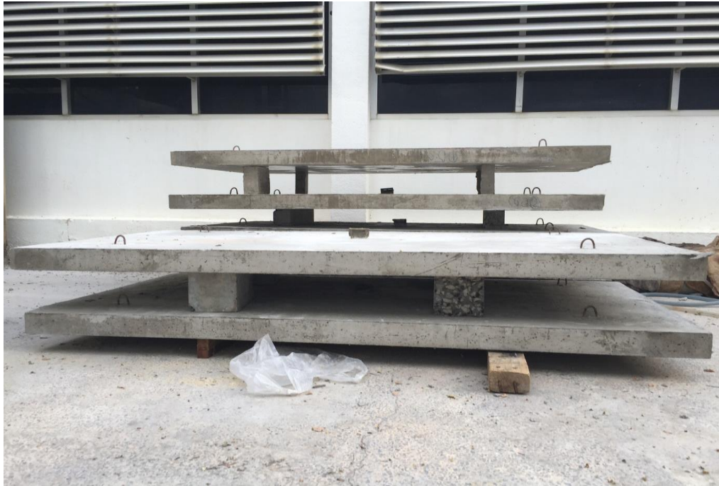
Figure 3.2-4 Wet cure and storage of casted panel
