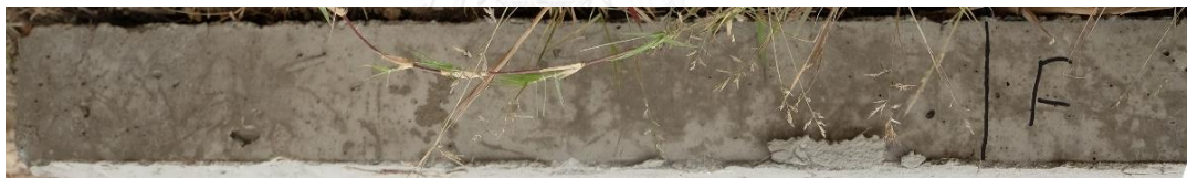
Figure 5.1.1-17 Marked location D to f of 30SF2LB
