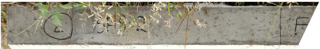
Figure 5.1.1-20 Marked location D to F of 60SF1LB
