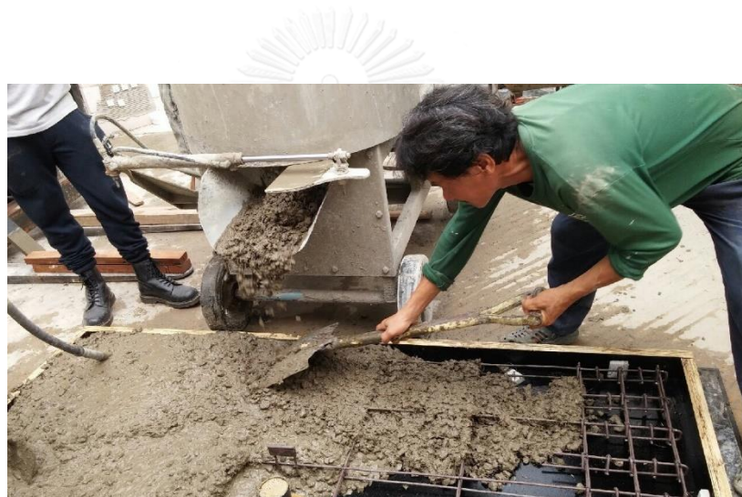
Figure 3.2-3 Casting of SFRC panels
