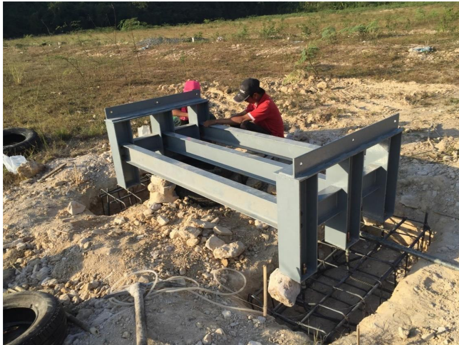
Figure 3.1-6 Steel cage in the foundation formwork
