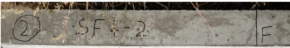
Figure 5.1.1-13 Marked location D to F of 30SF1LB
