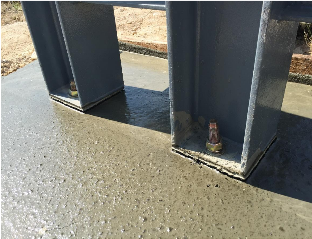
Figure 3.1-5 Bolted support after casting of concrete
