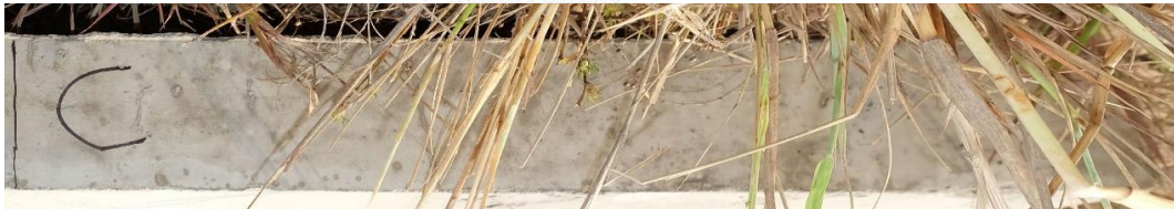
Figure 5.1.1-4 Marked location A to C of NRC1LB
