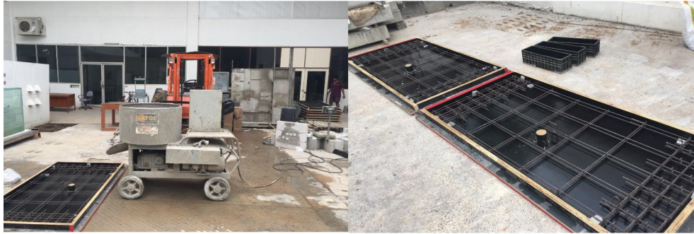
Figure 3.2-1 Form works and mortar mixer prepared at the site
