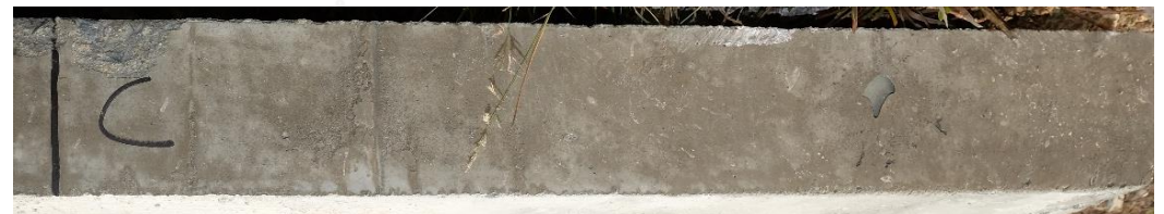
Figure 5.1.1-8 Marked location A to C of NRC2LB
