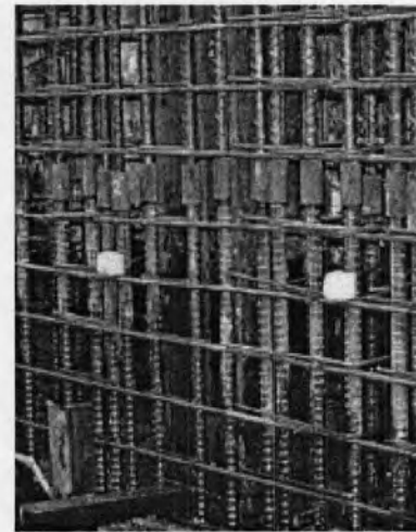
Shear Wall Application
