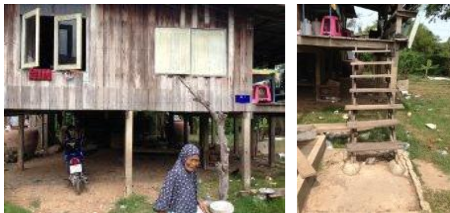
Figure 4.2: Some family chose to make use of compensation on improving the economic means rather than reconstructing destroyed structures. (Muslim Senior 1)
