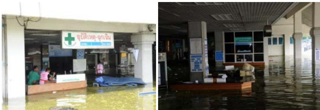
Figure 2.3: Flood water at Ayutthaya Hospital was as high as 2 m.
