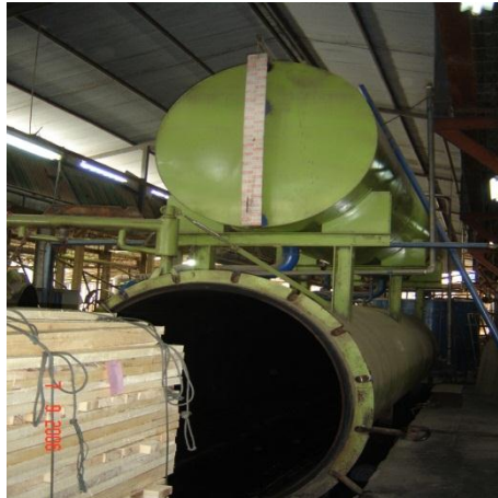
Figure 2.3 The planks were put into a vacuum tank for preservative
