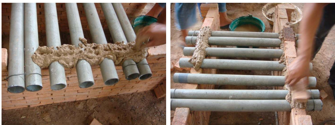
Figure173 Build brick masonry on the zinc pipe.
