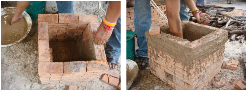
Figure 187 Plaster upper part of furnace with clay paste.
