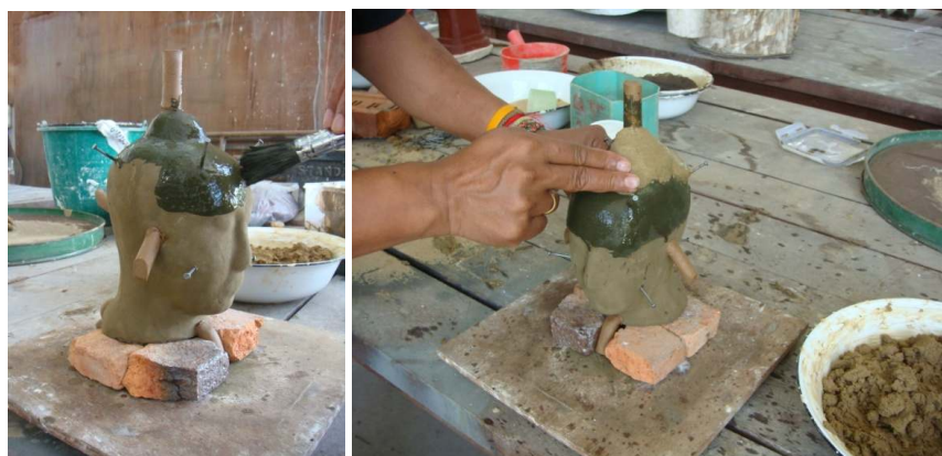
Figure 152 Apply cow dung and clay paste as glue and stick clay/ sand mixed plaster.
