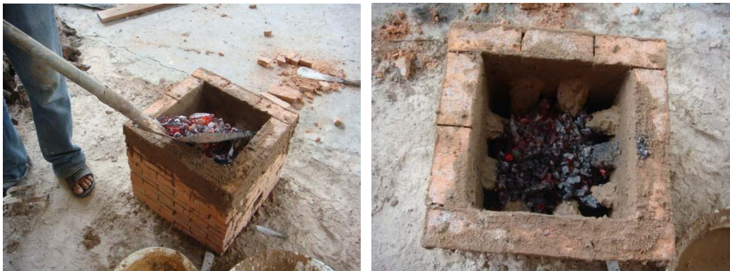
Figure191 Put burnt charcoal on the wet clay to dry faster.
