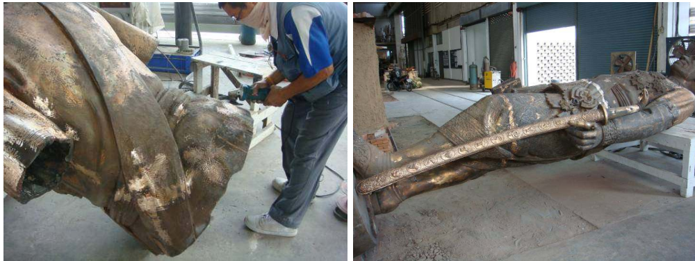
Figure 108 Grind uneven parts to make shine.
