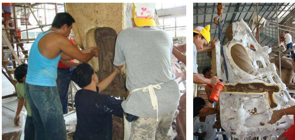
Figure 49 Separating plaster mould of the back of the seat.
