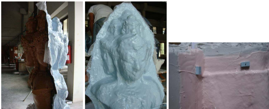
Figure 71 Apply Silicone Rubber on the thin cotton fabric.
