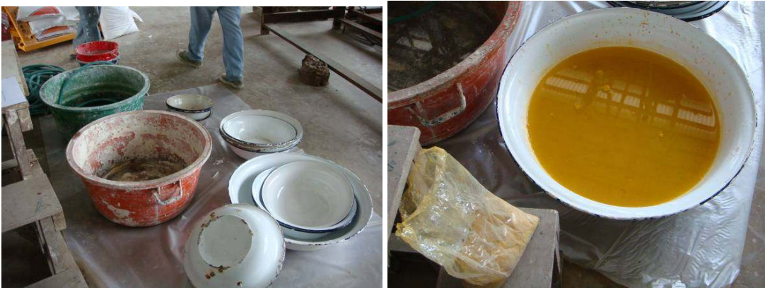
Figure 36 Mixture of Coconut oil and soap solution apply on the surrounding wooden surface.
