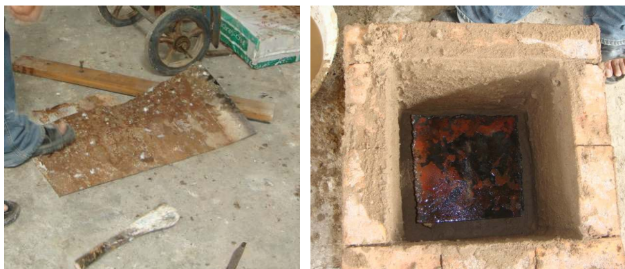
Figure 189 Place zinc sheet on the air circulation brick.
