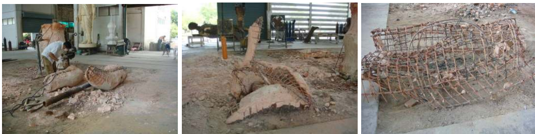
Figure 104 Cut out outer layer of plaster and iron strengtheners.
