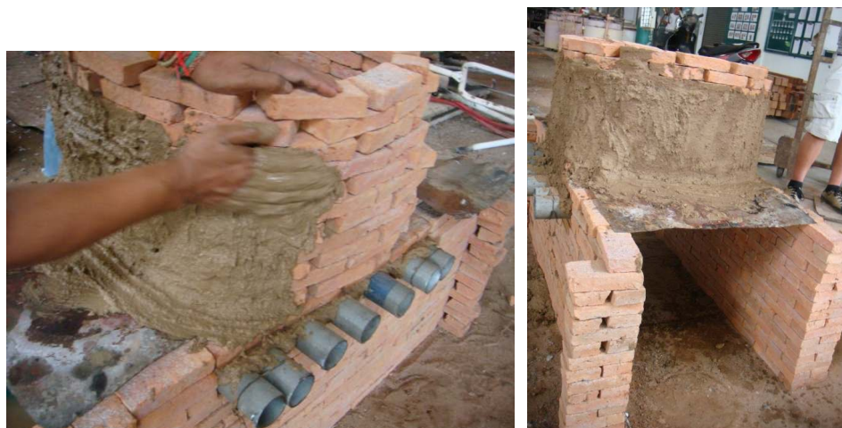
Figure175 Apply clay and sand mixed plaster on the brick wall.
