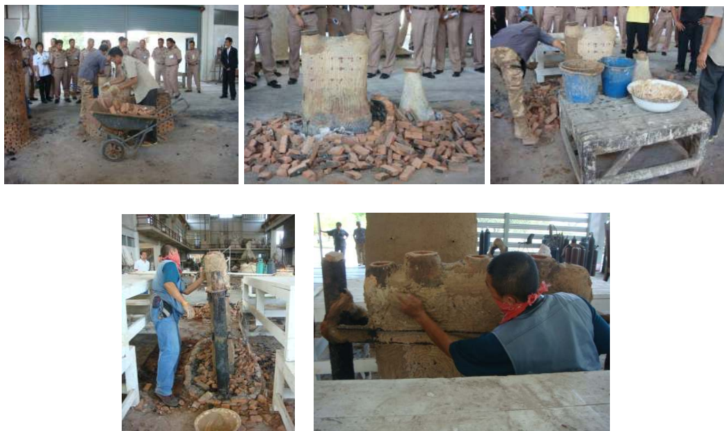
Figure 94 Dismantle surrounding brick wall and close possible holes with wet clay plaster.
