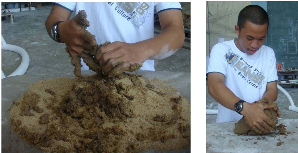
Figure 124 Mixing sand and wet clay.
