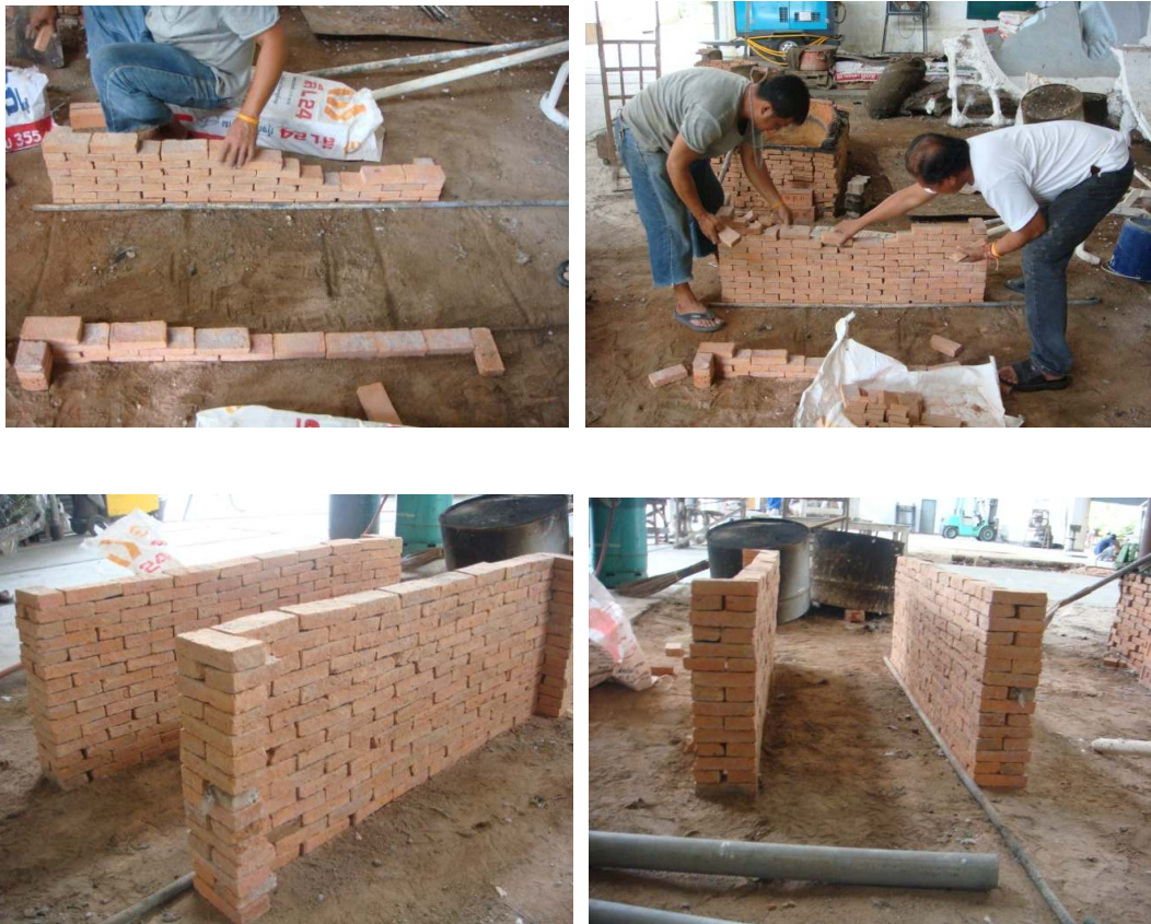
Figure171 Constructing Kiln with brick.
