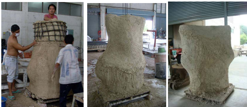
Figure 88 Applying Gypsum plaster and sand mixed plaster on the iron frame.
