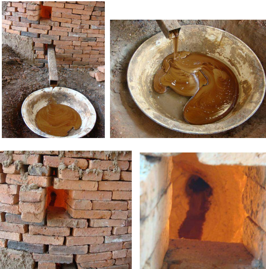
Figure 91 Wax running out from pipe and tiny hole to see the status of wax running out.
