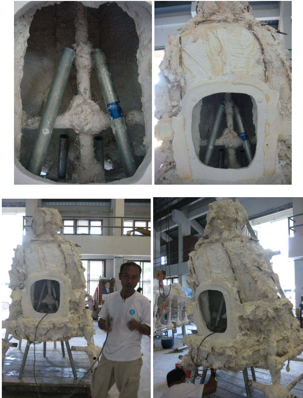
Figure 61 Strengthen and join zinc pipe to make stand for the mould.
