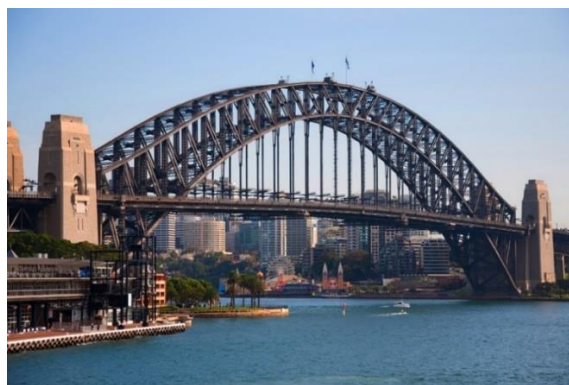
Fig . 2.1 Sydney Harbor Bridge (503 m, year of completion 1932), Sydney.
