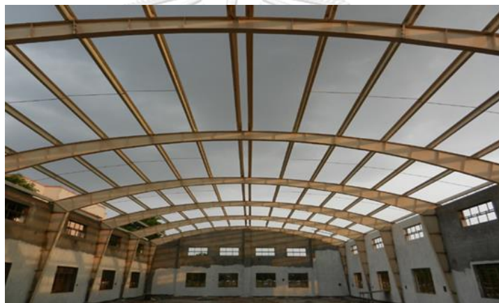
Fig . 1.3 PEB arched clear span.
