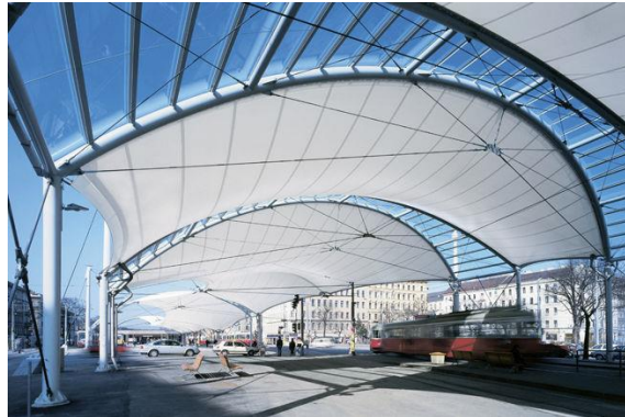
Fig . 2.2 Urban Loritz Platz (130 m, year of completion 2000) , Vienna, Austria.
