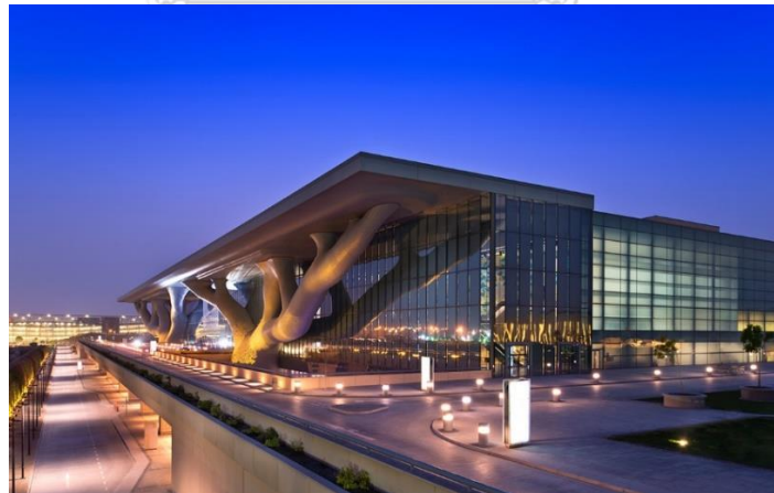
Fig . 4.1 The Qatar National Convention Centre ( http://www.amlak.com.qa ).
