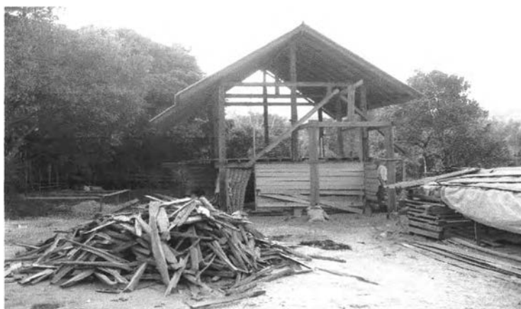
Figure 2.6.4: Constructing a house
