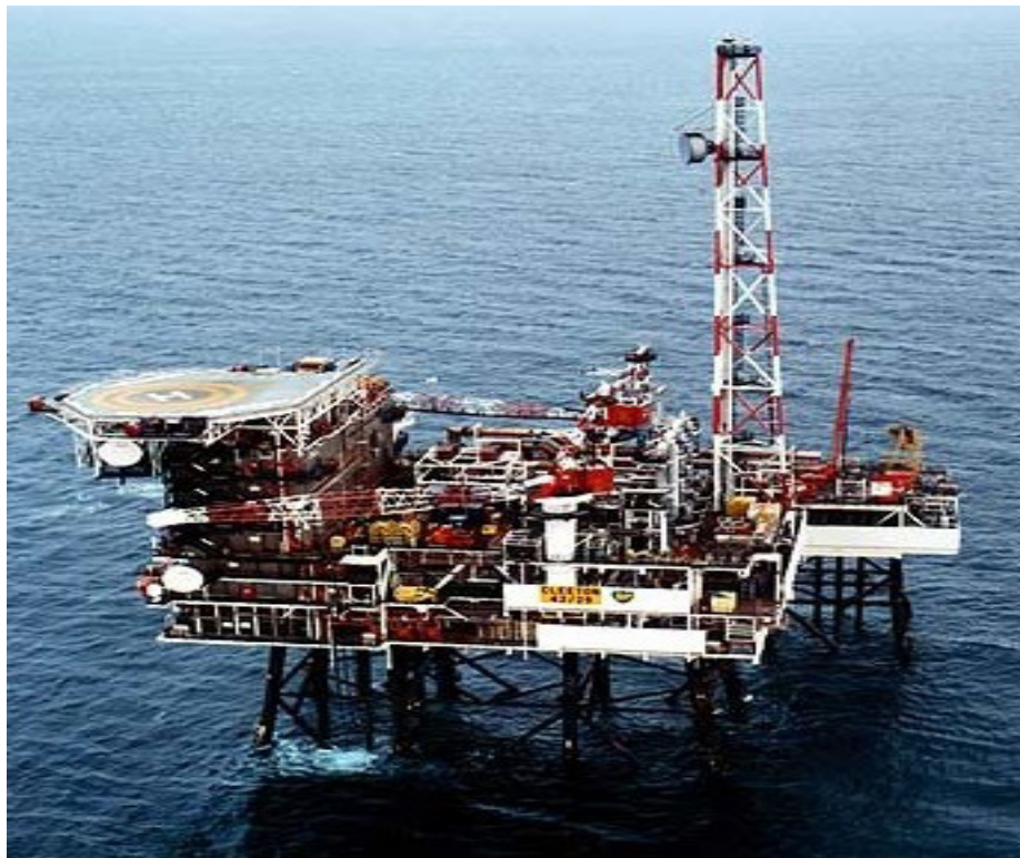
Fig 3: Steel jacket platform rig (www.planete-tp.com)
