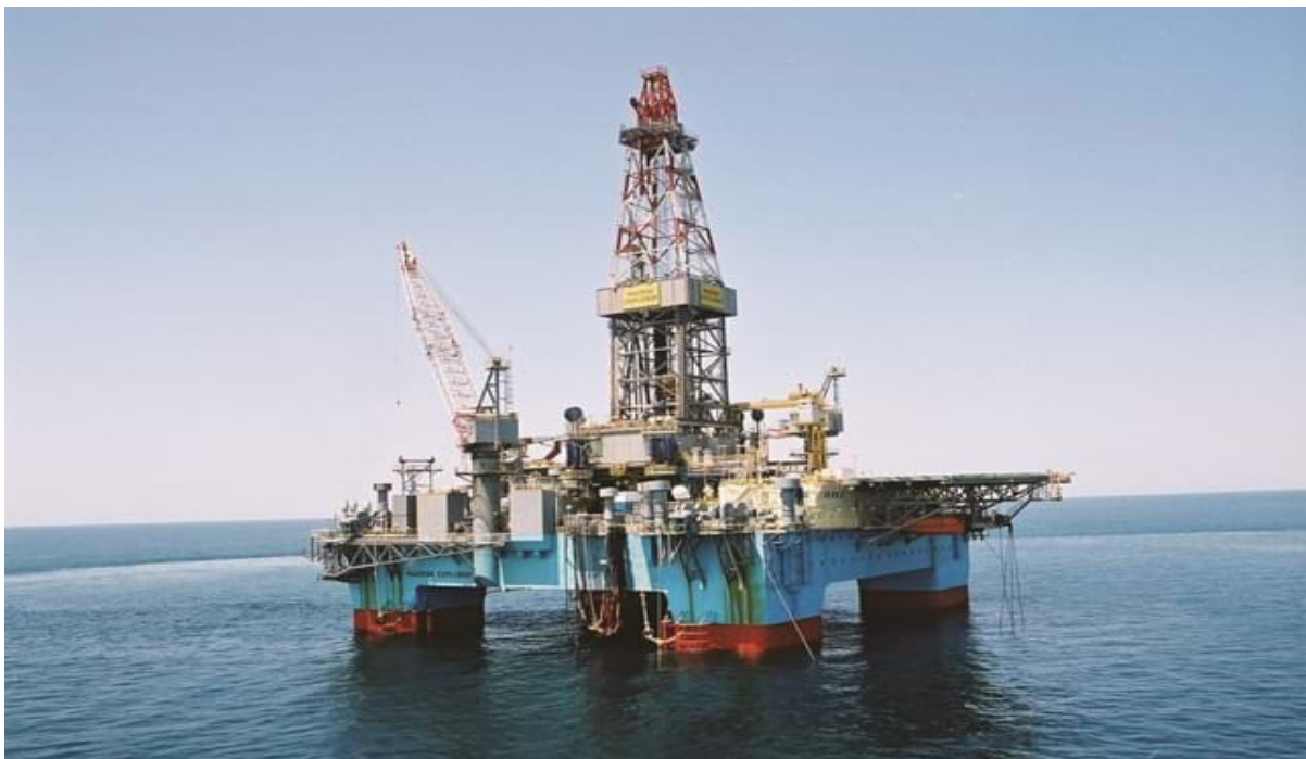
Fig 8: Semisubmersible rig (www.maerskdrilling.com)
