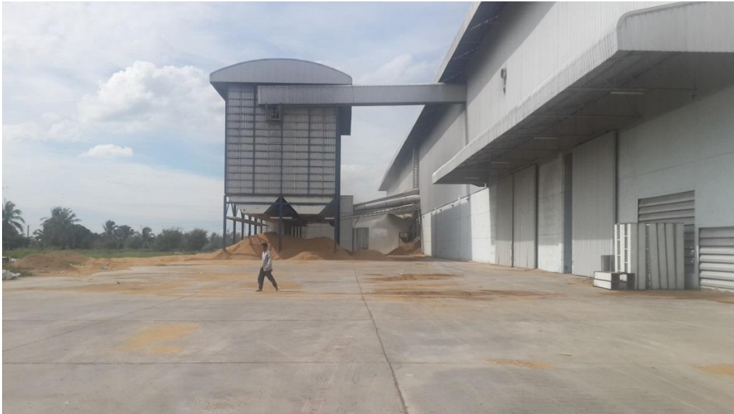
Figure 3-3View of rice husk storage area
